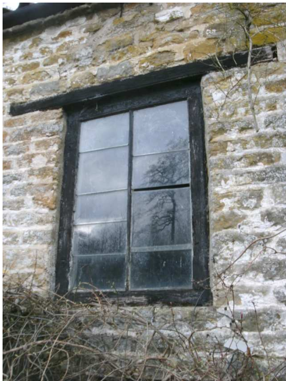
window, with lapped panes of glass
