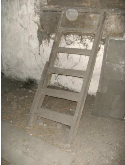
door into attic of house from within millhouse
