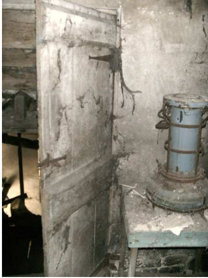
one of double doors between house and mill-house attics
