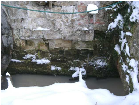
high status ashlar of lower mill-house wall (left), much frost-damaged. Higher status sandstone to right of doorway of mill-house (below).
