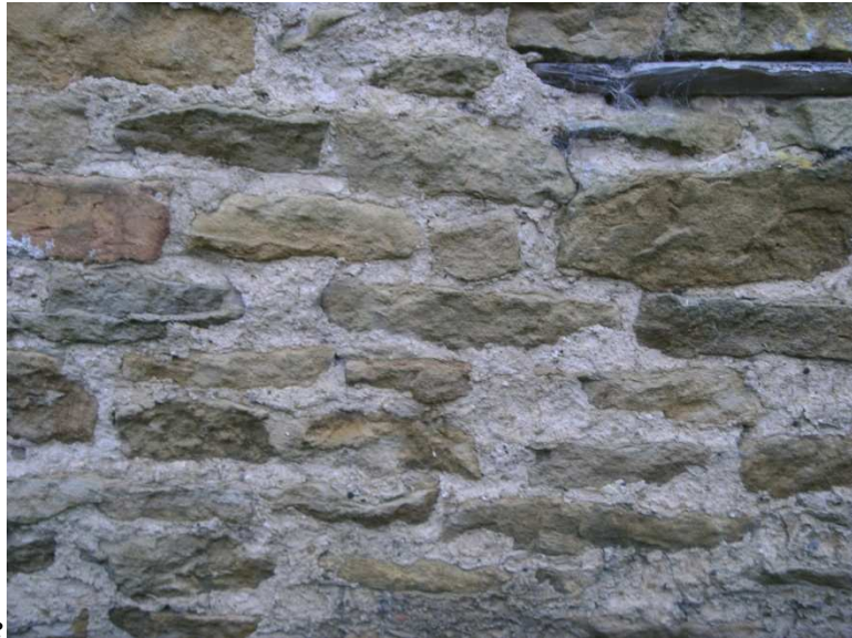
lime pointing, cow byre
