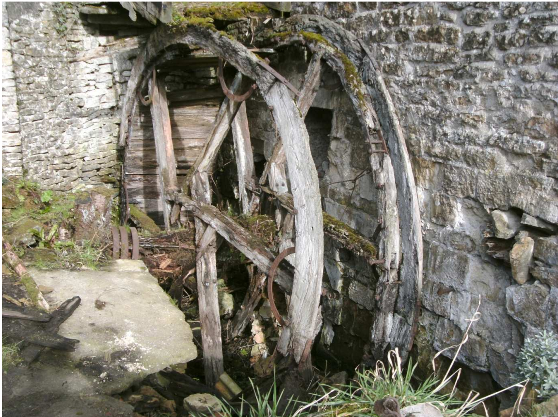
part of the mill dam. The buttress of this is battered, not leaning; the retaining wall of the tail-race is at left and returned along the line of the back wall of the pig-sheds and forge, they being part of the same retaining wall.
