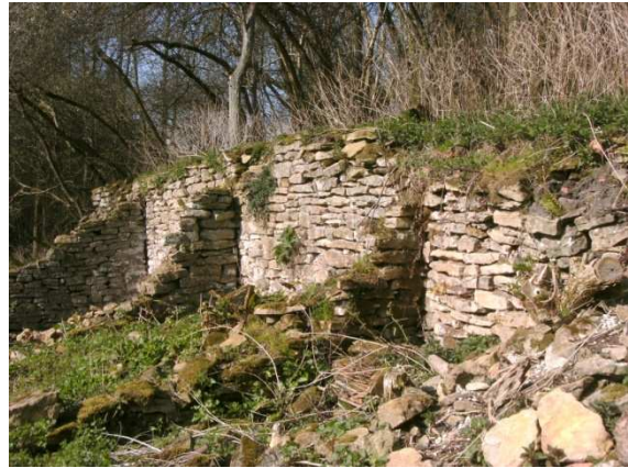
junction of mill-dam and forge walls (below), the former returning S as part of the rear wall the pig sties (left).
