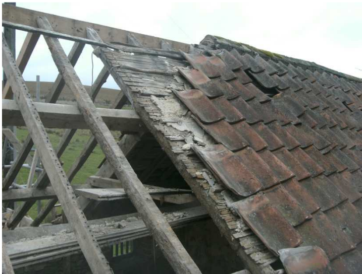
lime 'sheeted' roof of cow byre
