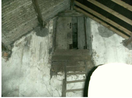
ladder to the above. This doorway and the one within the two-bay attic are wide, indicating their storage purpose
