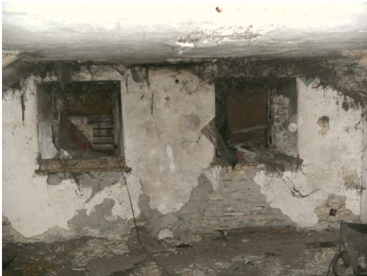
blocked windows, N end
