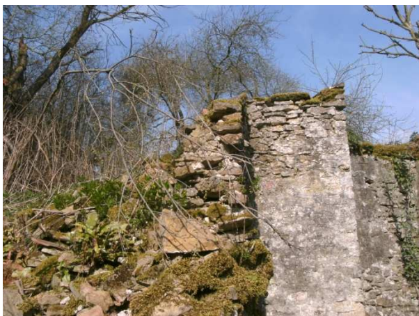
part of the mill dam. The buttress of this is battered, not leaning; the retaining wall of the tail-race is at left and returned along the line of the back wall of the pig-sheds and forge, they being part of the same retaining wall.
