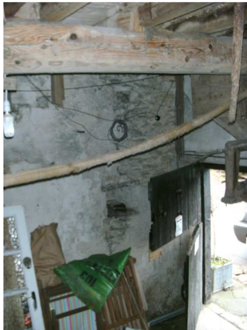
Inside of mill-house
