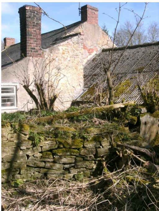
stone wall of the head-race as it turns to feed the pentrough (left) and tail-race (below).
