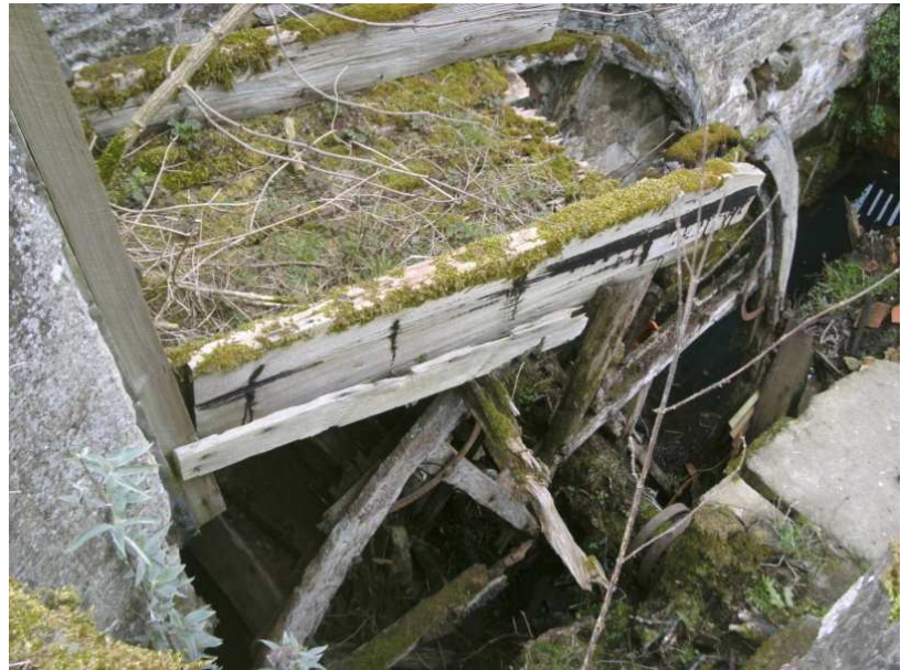
the trough and wheel, with remnant penstock at left of picture
