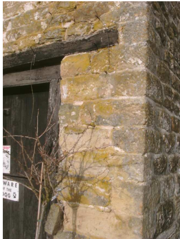
high status ashlar of lower mill-house wall (left), much frost-damaged. Higher status sandstone to right of doorway of mill-house (below).
