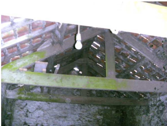
truss over single storey loose-boxes
