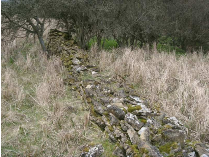
dry-stone wall of the former 'fold-yard'.
