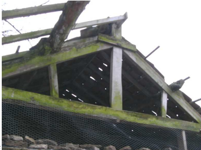
truss over single storey loose-boxes
