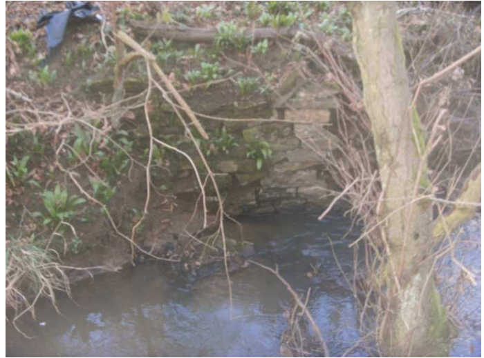
part of the sluice at the onset of the mill leat
