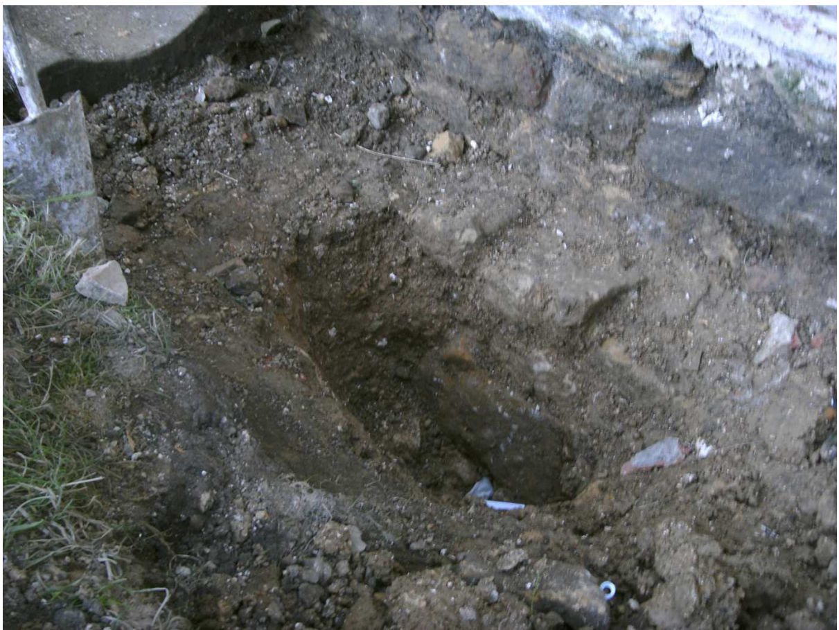
Stone footing of N channel wall beneath this channel stone
