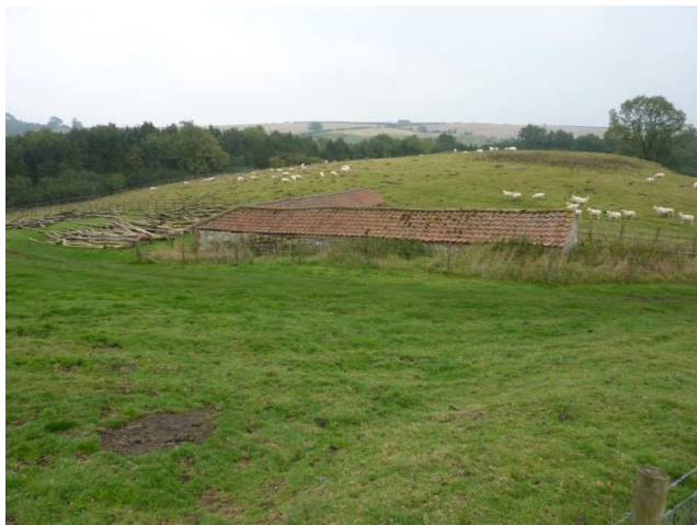
looking south across the site
